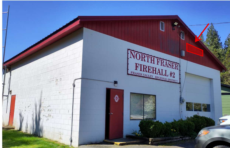
Figure 6: Recommended Exhaust Louvre Outlet Location
