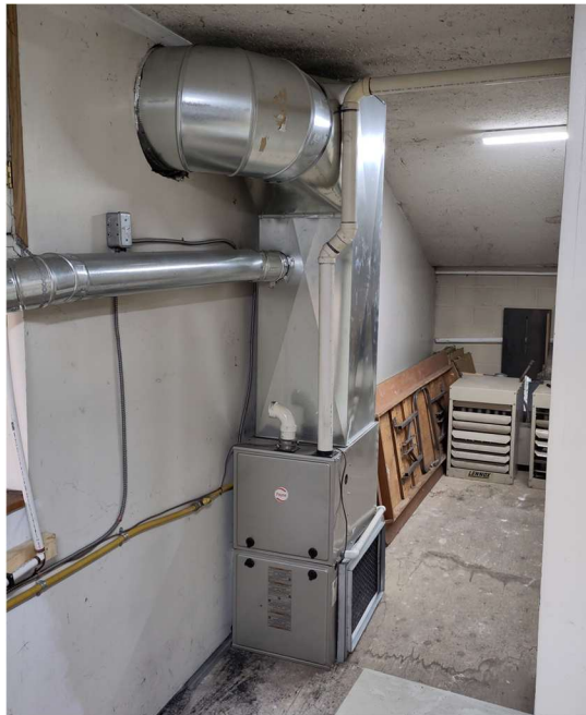
Figure 1: Hall #3 Natural Gas Furnace (75,000 btu/h)
